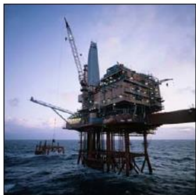
Crude Oil Exploration & Production
