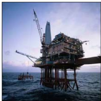
Crude Oil Exploration & Production
